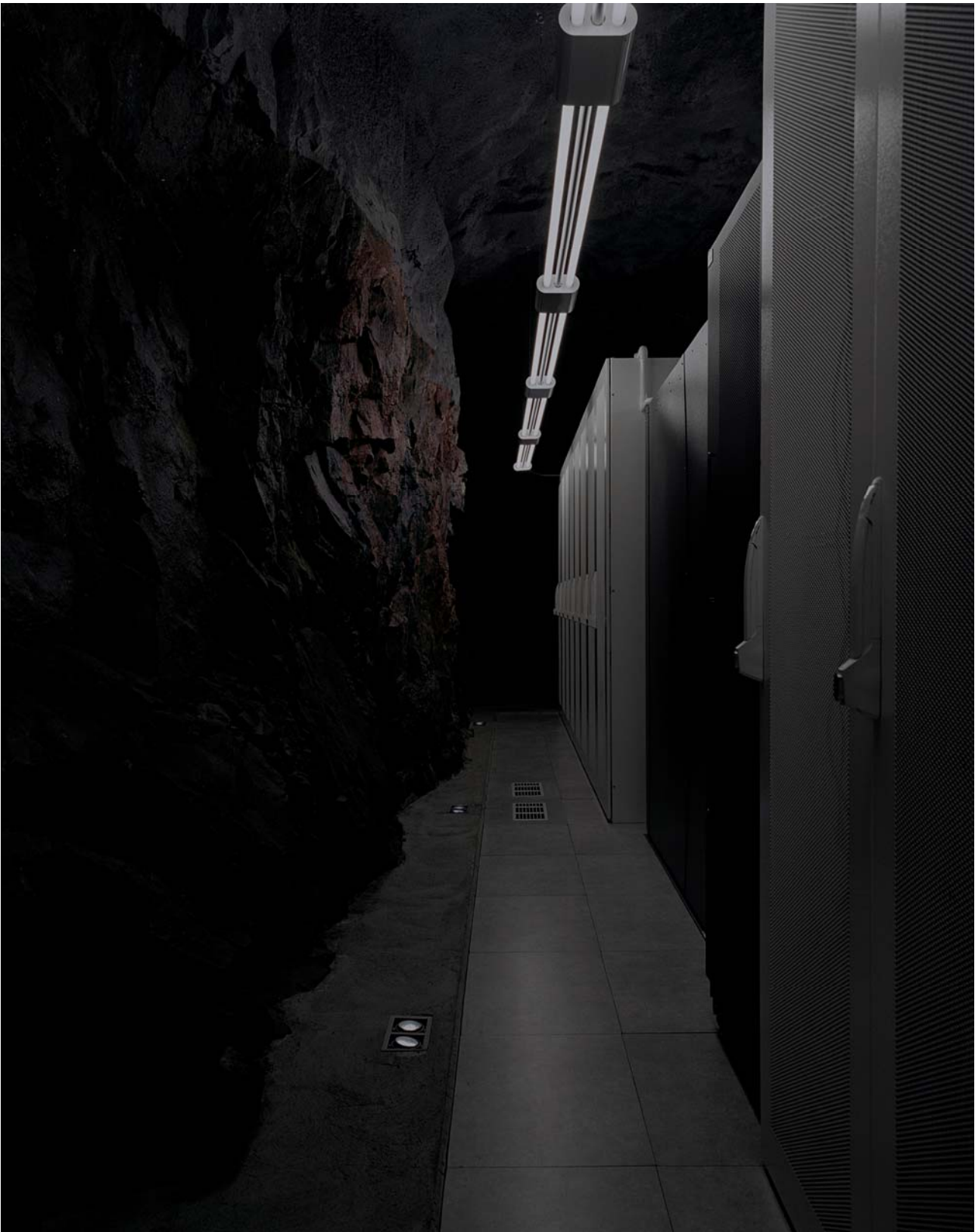
© Yann Mingard, Bahnhof.se , "Pionen" High security computer centre, Stockholm, 2011, Deposit Series , pigment print, 70x55.4 cm. Main room hewn into the rock.
